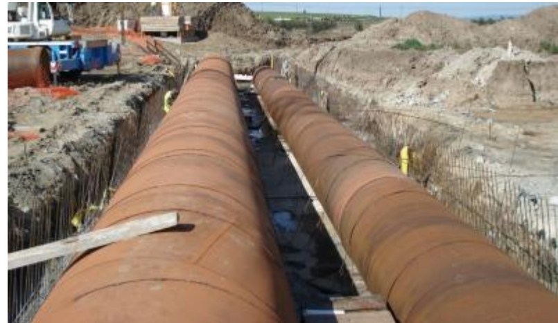
Detail of reservoir pipes – EDIA | Portugal
