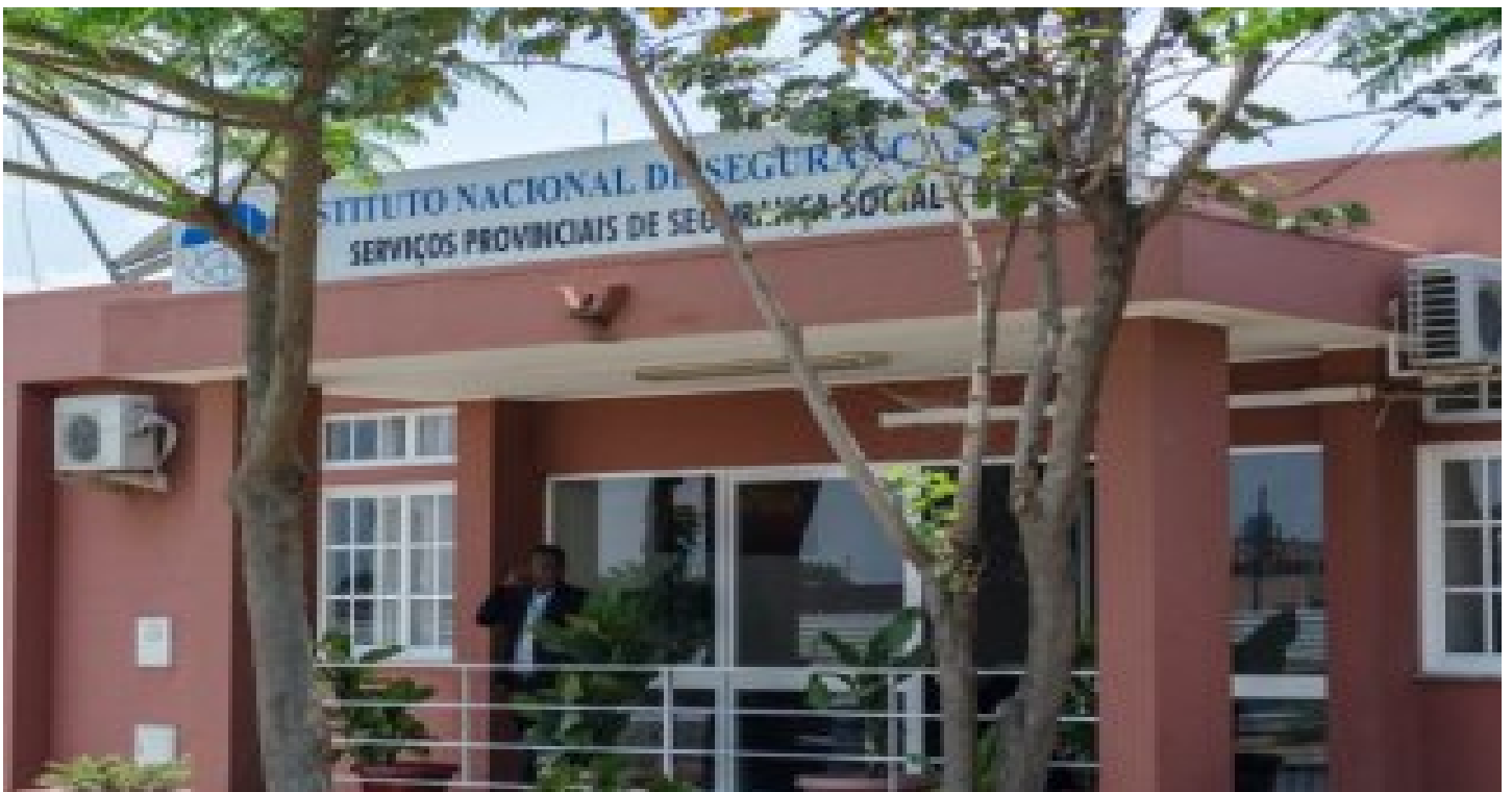
MAPESS and INSS Provincial Buildings
