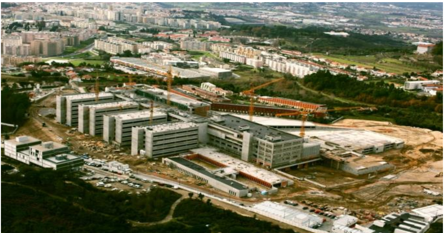
Novo Hospital de Braga
